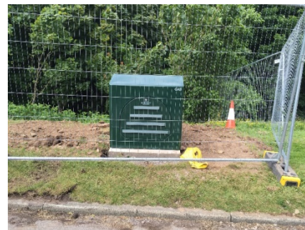
13b New gas meter housing
