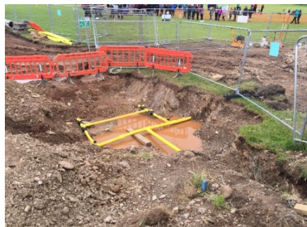
13a New Gas main installed
