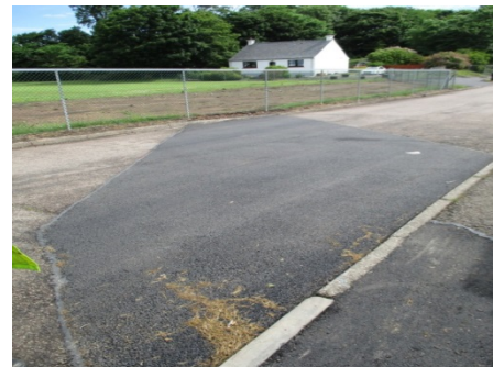
8 Re-instatement of Limecraigs Road
