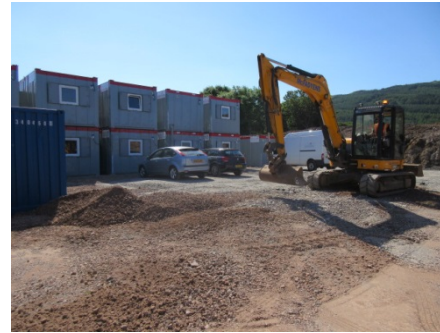
4 Site compound offices
