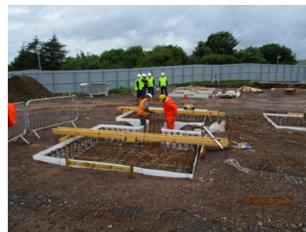
15a Preparing Concrete Foundations
