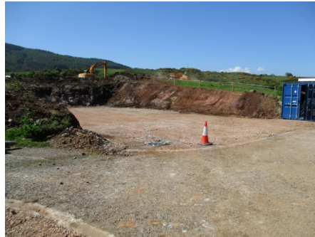
3 Site compound area
