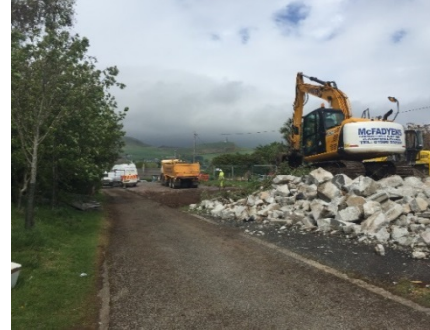
11b Demolition of the Boat Shed
