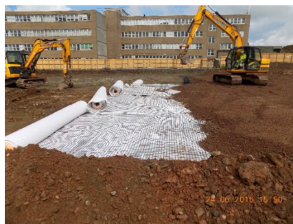
14 Preparatory ground works
