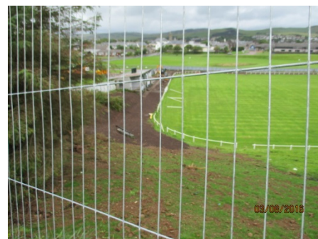
10 Kintyre Park re-instated following culvert works
