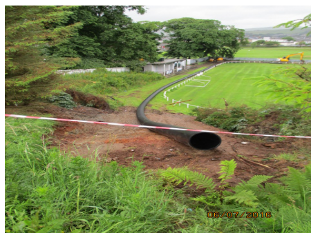
9 Culvert pipe within Kintyre Park
