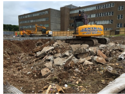
12b Music Block demolition
