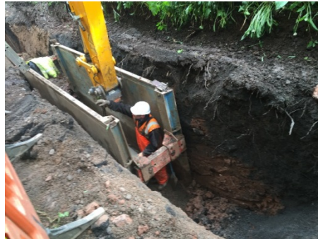
5 Culvert works taking place in the Cutting
