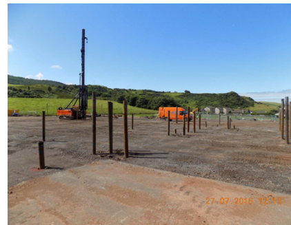
16b Piling works
